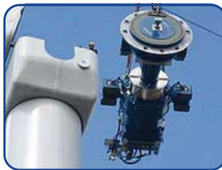
Figure 3-11. Typical components of a wind turbine (the gearbox, rotor shaft and brake assembly).
